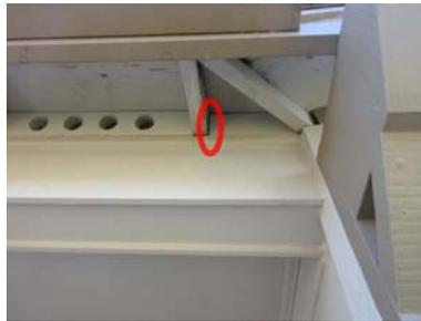
The beams that stick out beyond the drip edge of the roof are vulnerable to rot damage. They should be covered with a metal cap flashing or cut off flush with the edge of the overhang.
